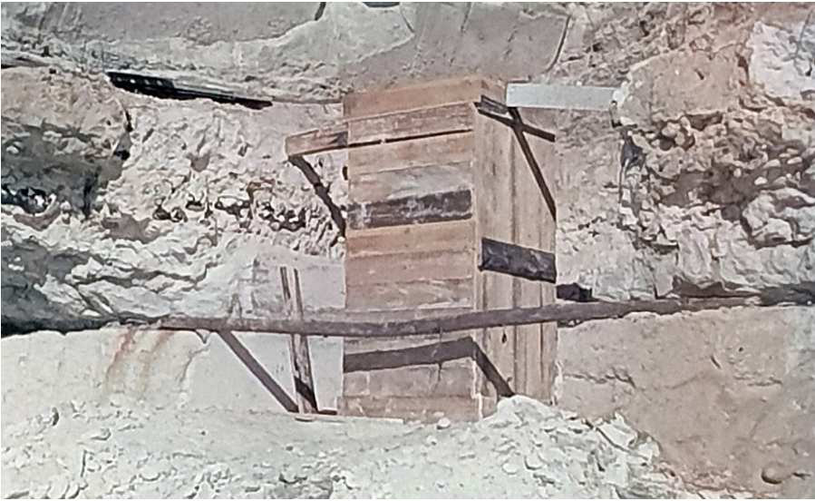
Fig. 8. The column sawn completely free, packed in a case of wooden boards and ready to be hoisted to the top of the cliff.
