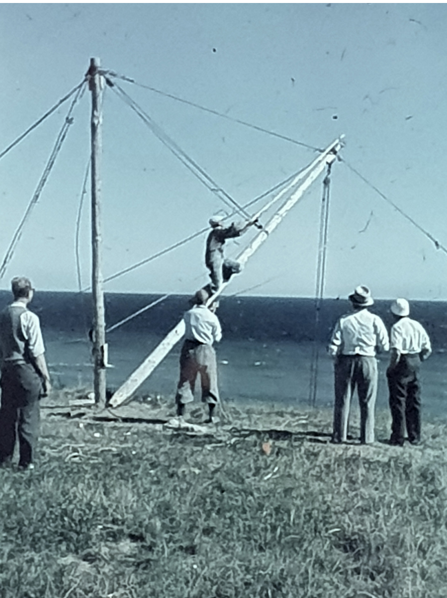
Fig. 9. A simple crane was constructed at the cliff top.
