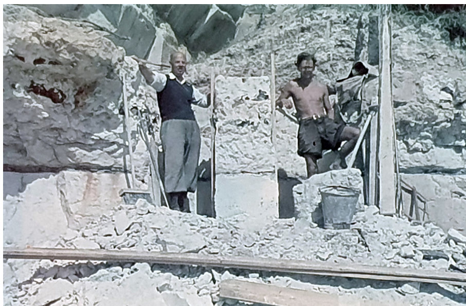
Fig. 7. The column almost free, only the base needed to be sawn and the wooden board to the right ready to be packed around the column.
