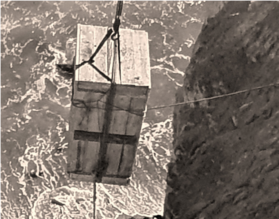
Fig. 10. Start of lifting the column to the flat surface at the top of the cliff.
