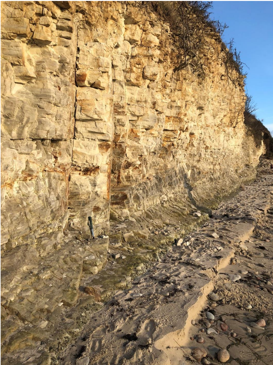
Fig. 6. Two closely associated, near-vertical and through-going fractures. The fractures are trending W–E; hammer at base of the cliff for scale. Cliff is viewed from the west. Picture taken at evening Sun.
