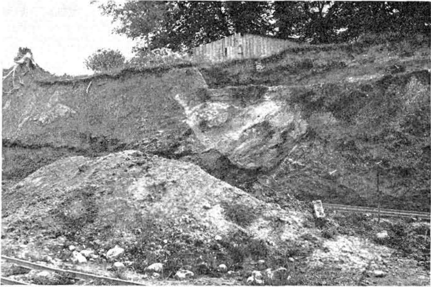
Fig. 7. The clay pit in the esker-like ridge at Katrinedal brickworks. In the middle of the sequence a large ball of sand in the clay is seen.
